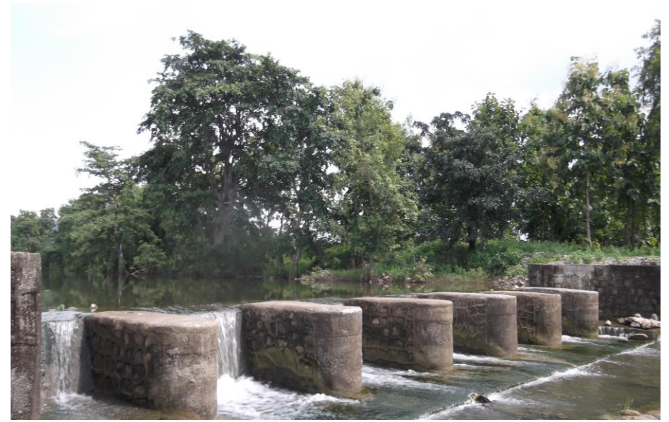
constructing check dams
